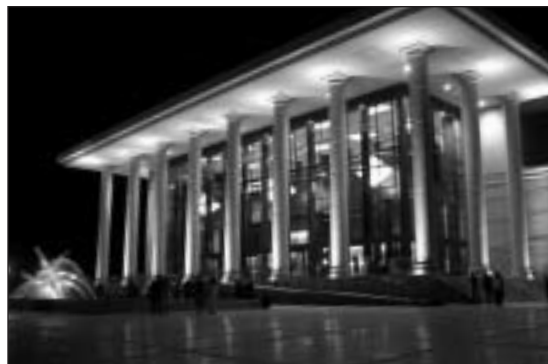
Armstrong Auditorium, Edmond, Okla., at night
