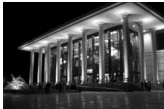
Armstrong Auditorium, Edmond, Okla., at night
